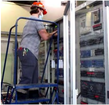
Removing Relay (Replacement)
