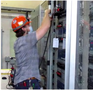
Connecting Test Equipment
