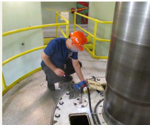
Checking Turbine Oil Level
